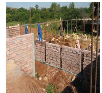
Facility under construction in São Leopoldo, RS, Brazil
